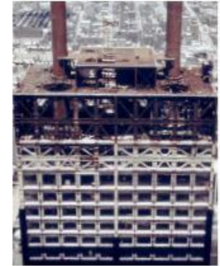
Figure 4. Gravity load transfer through belt truss
