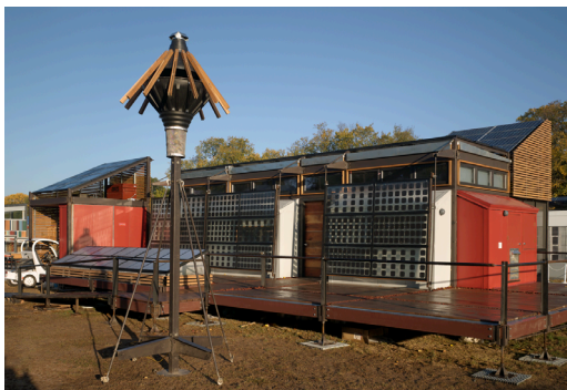
Figure 10. Constructed "groHome" (photo by College of Architecture)
