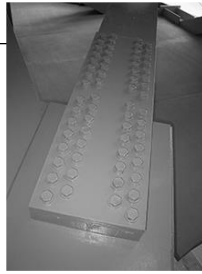
(AISC - Steel Structures of the Everyday)
